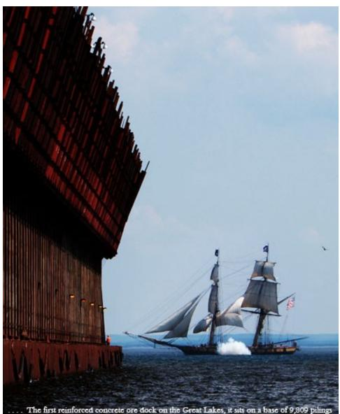
of Oregon fir driven 20 feet into the lake bottom. A 9-ft. thick cap of reinforced concrete tops the pilings, making a foundation that has endured 100 years of vibration from train engines and ore cars.
