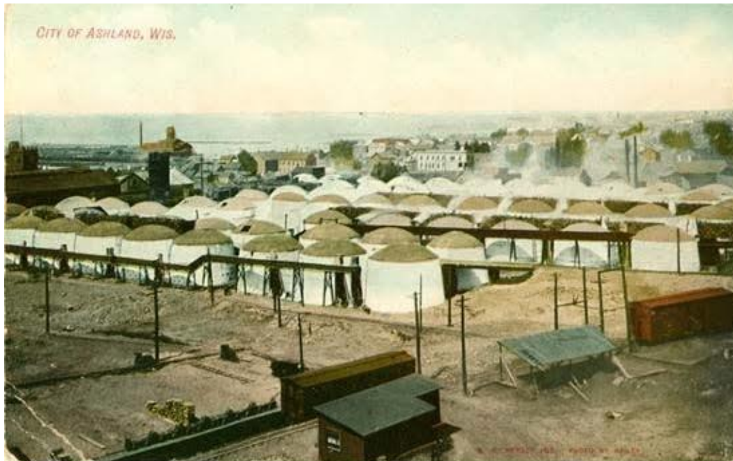
Figure 4. Round charcoal kilns at the Ashland Iron and Steel Company, Ashland, Wisconsin. Note the vertical sides and arched tops. Round kilns tended to be in batteries near the furnaces or at railroad locations. (Image courtesy of Ashland Historical Society Museum.)
