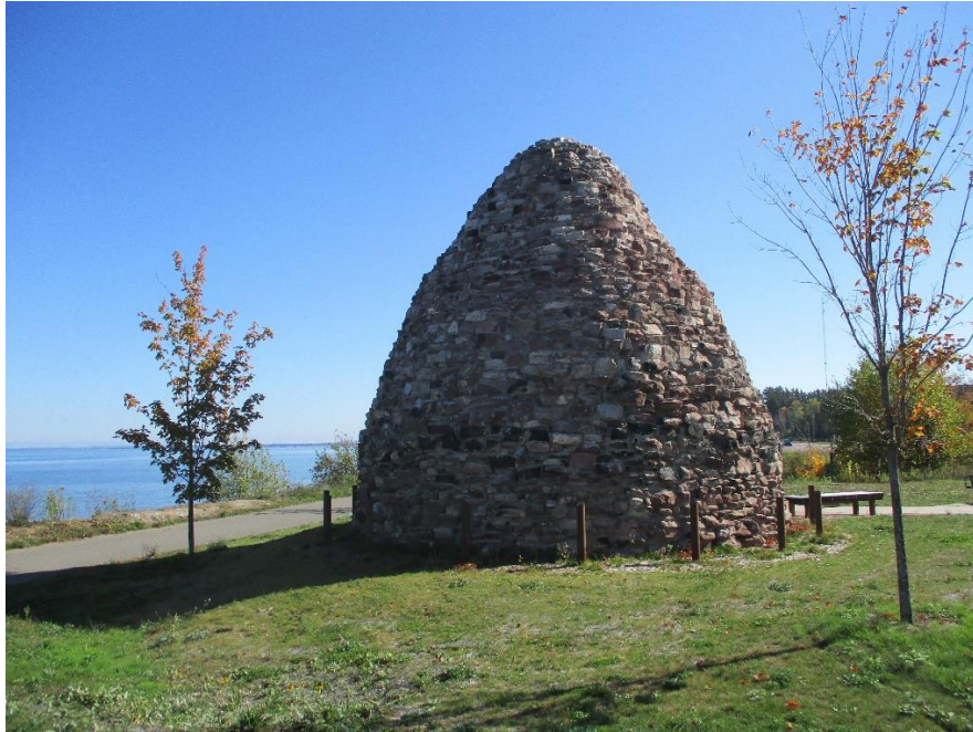
Figure 5. BEEHIVE CHARCOAL KILN. The reconstructed Marquette kiln with the beehive design, somewhat conical as it tapers upward, and with a parabolic dome. This kiln is on U. S. Highway 41 South where it crosses the Carp River. (Image by author.)
