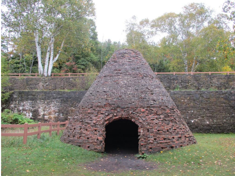
Figure 6. CONICAL CHARCOAL KILN. The reconstructed charcoal kiln at the Fayette Historic Townsite has a conical shape without a parabolic dome. (Image by author.)
